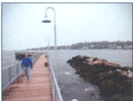
Rebuilt pier opens at Cummings Beach
